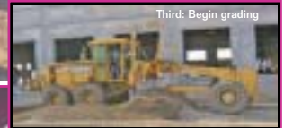
Third: Begin grading
