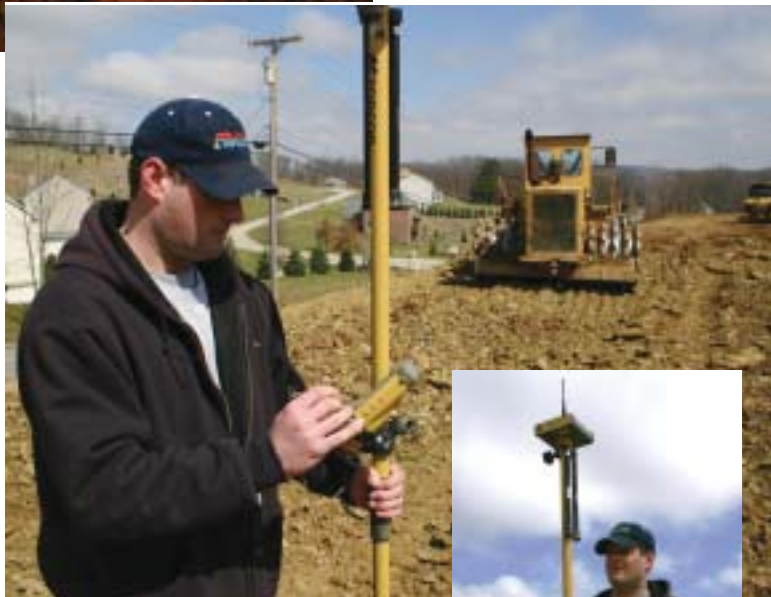
Jim McGowan of McGowan-Stauffer Inc. checks grades with Topcon's HiPer+ survey system to analyze the site for design adjustments.
